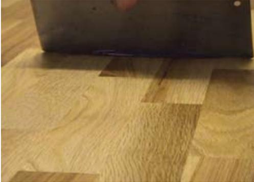
Step 6. The second coat is applied in the same manner as the first using a scraper to spread the material over the floor.
