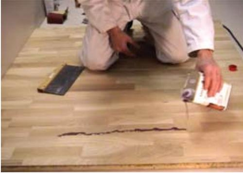
Step 1. Pour the finish directly onto the properly prepared floor.
