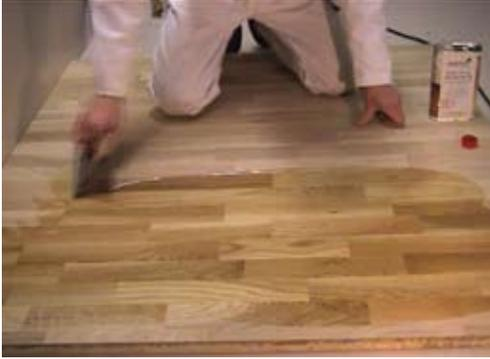
Step 3. Pull the finish over the floor 4-5 times before moving onto the next area.
