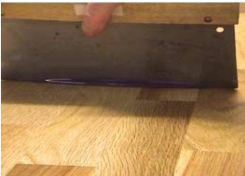
Step 2. Spread the finish over the floor using a metal blade, such as the Osmo pro scraper.
