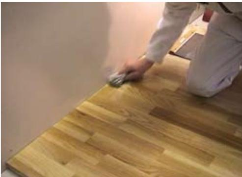
Step 4. For edge detail and hard to reach areas use a cloth to apply the finish.
